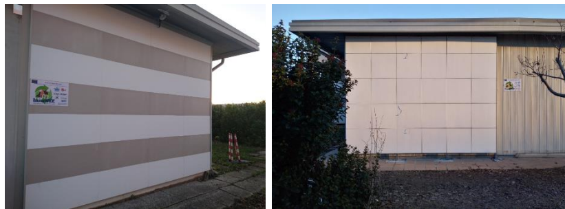
Fig. 1: ETICS-like (left) and ventilated façade (right) geopolymer panels, installed in the Padova demo-site
